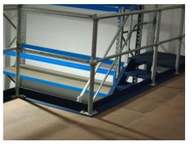
Handrails and kickplates provide a level of fall protection and safety to other users.
