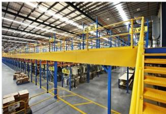
A raised platform made from structural steel is so strong you only need a limited number of pillars.
